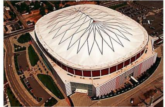
The roof of the “Georgia Dome” in Atlanta, Georgia can be considered as a thin membrane.
