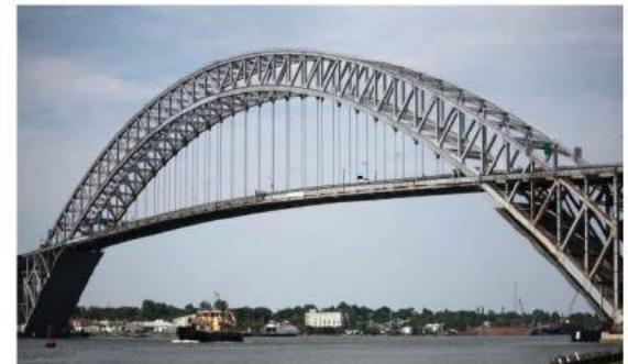
Arches support their loads in compression
