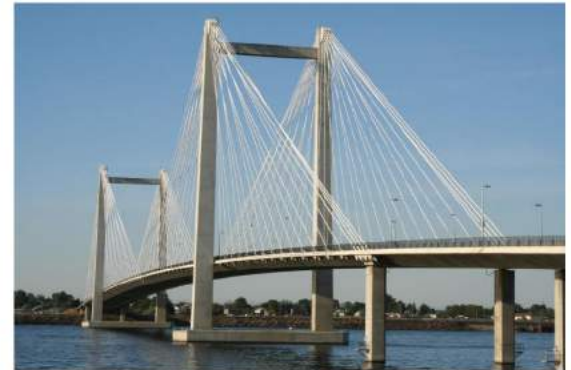
Cables support their loads in tension.
