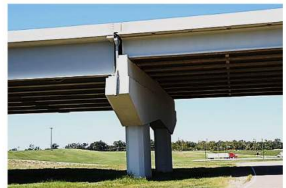
The prestressed concrete girders are simply supported
